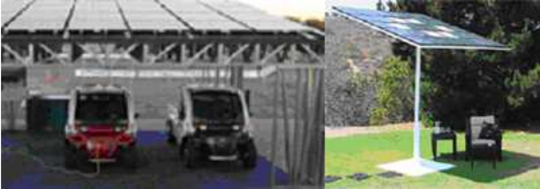
Figure 4 – a lightweight steel frame Envision Solar 2.4 kW off-grid PV system charging two NEVs at an amusement park. An Envision 1.4kW Solar Tree is a great shade-maker.
